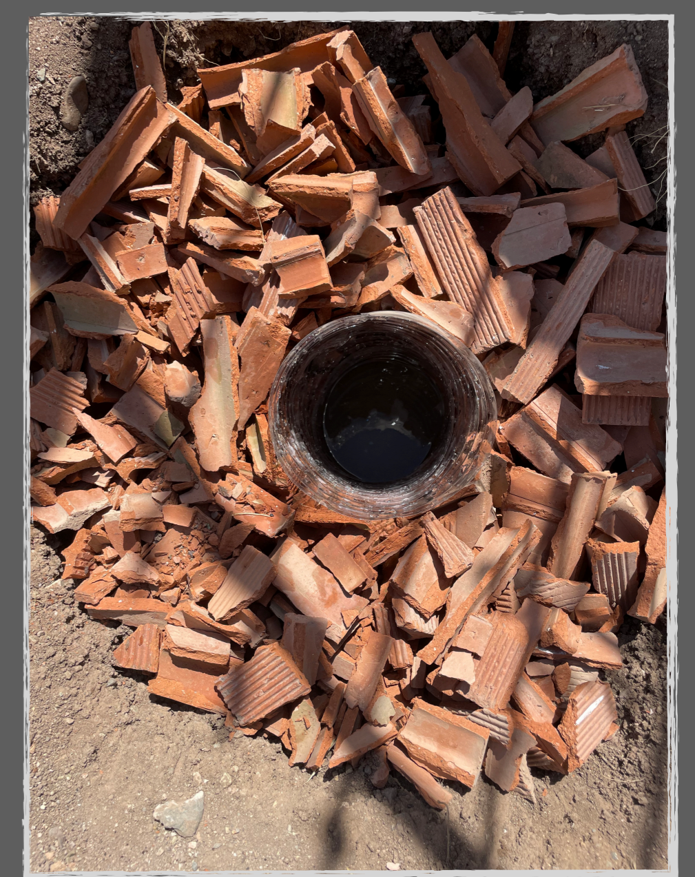
FIG. 3: RECONSTRUCTED SOAKAWAY WITH BRICK FILL
