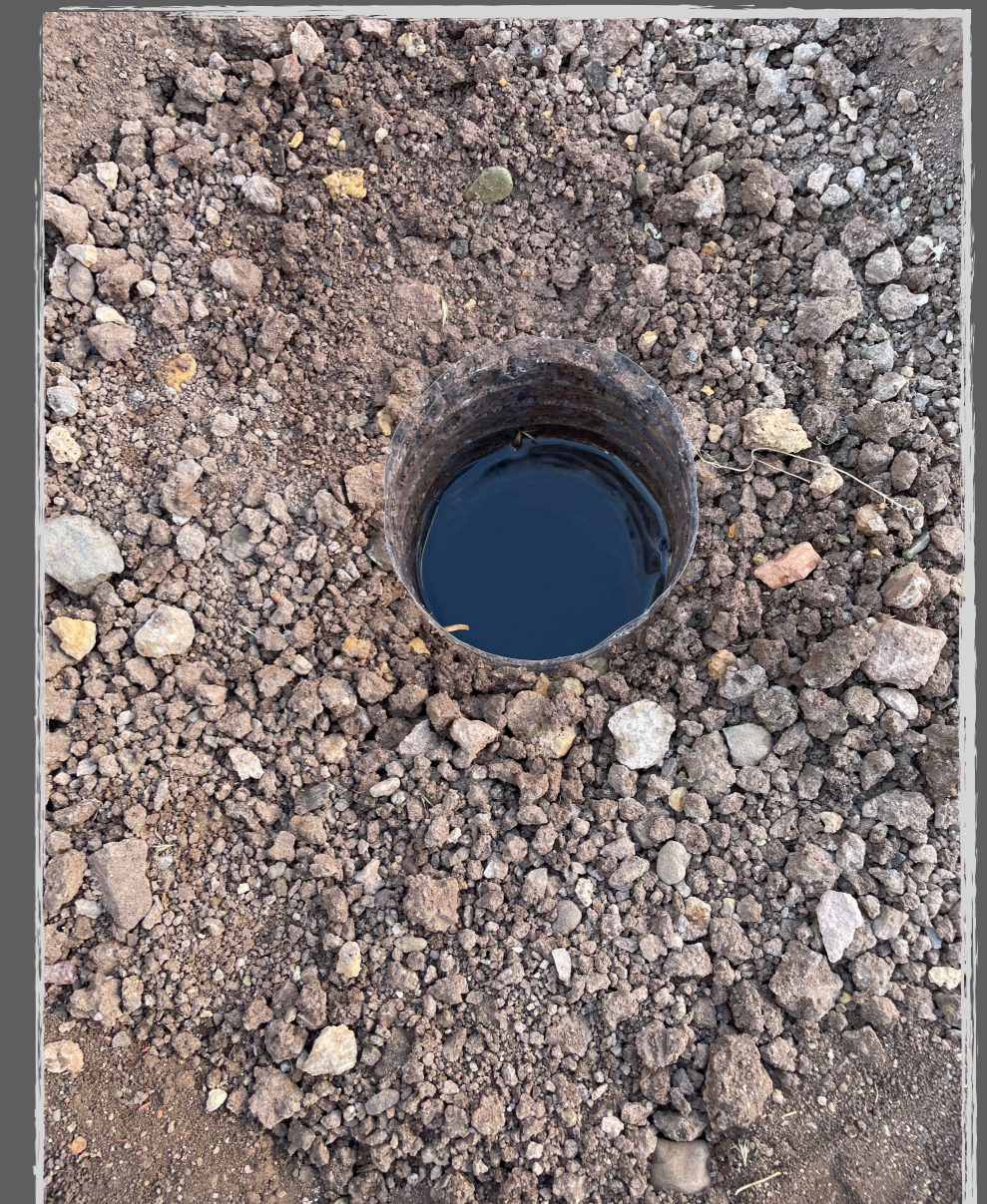
FIG. 4: RECONSTRUCTED SOAKAWAY WITH SOIL FILL
