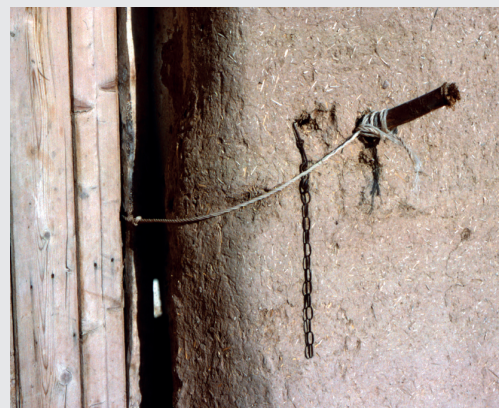
Fig. b. Modern “bolt” in a house of Tell Ahmar. A device similar to the ancient locking system is still in use in some houses of the village.
