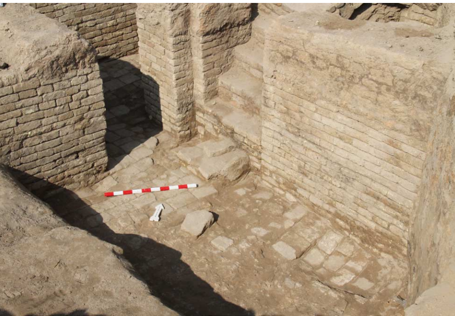
Figure 18. Staircase in House of Abisum. Note courses of unbaked mud bricks on top of fully preserved back brick courses. Photograph by Paul Zimansky.
